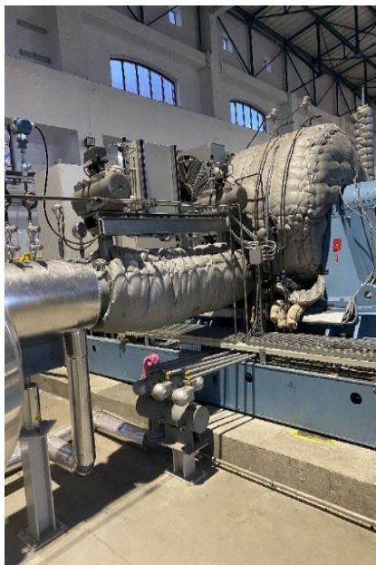
Fig. 1. Steam turbine in the chemical factory.
